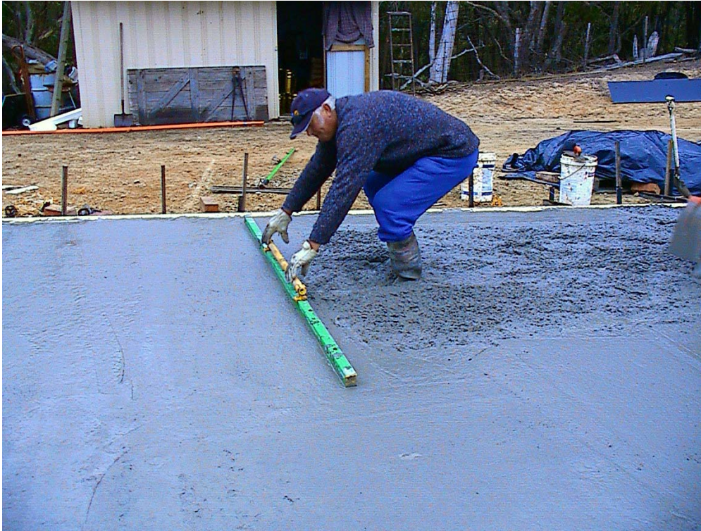
Figure 9 - Screeding off the First Commercial Slab of 80 Cubic Metres
