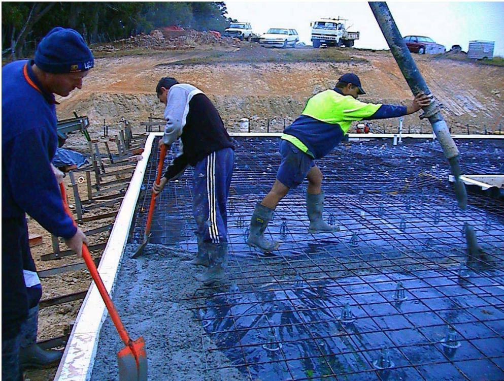
Figure 8 - Pouring the First Commercial Slab of 80 Cubic Metres
